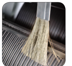
扶梯导静电装置 Handrail anti-static device
